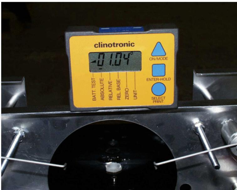
Then the digital clinometer is placed on the control plane in the light direction, and the ball joint on the back leg is adjusted to the desired angle for each individual PAPI light unit. Be careful not to touch the housing during the adjustment as angle adjustment is very sensitive.
